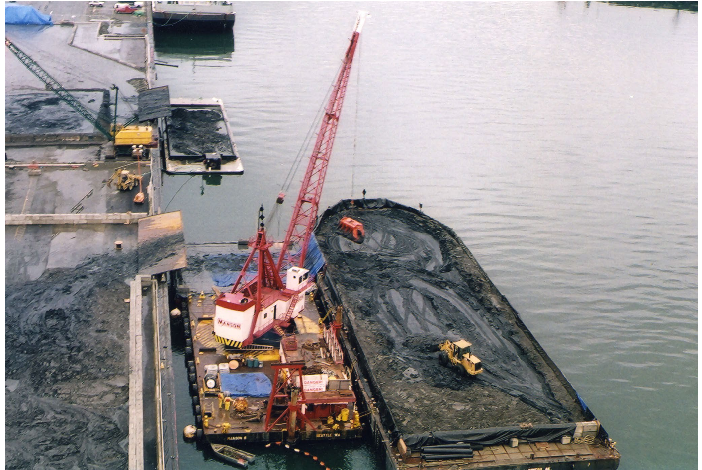
Offloading dredged material with closed bucket and spill aprons
