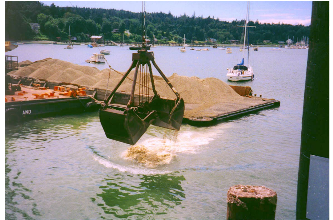
Placing material with open bucket
