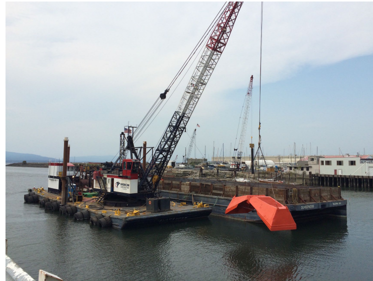
Derrick Barge with wireline bucket
