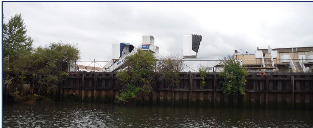
River Mile 3.8 East B – next to Area 18
