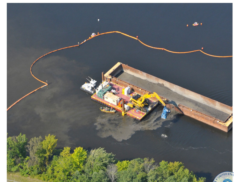
Hydraulic excavator and barge
