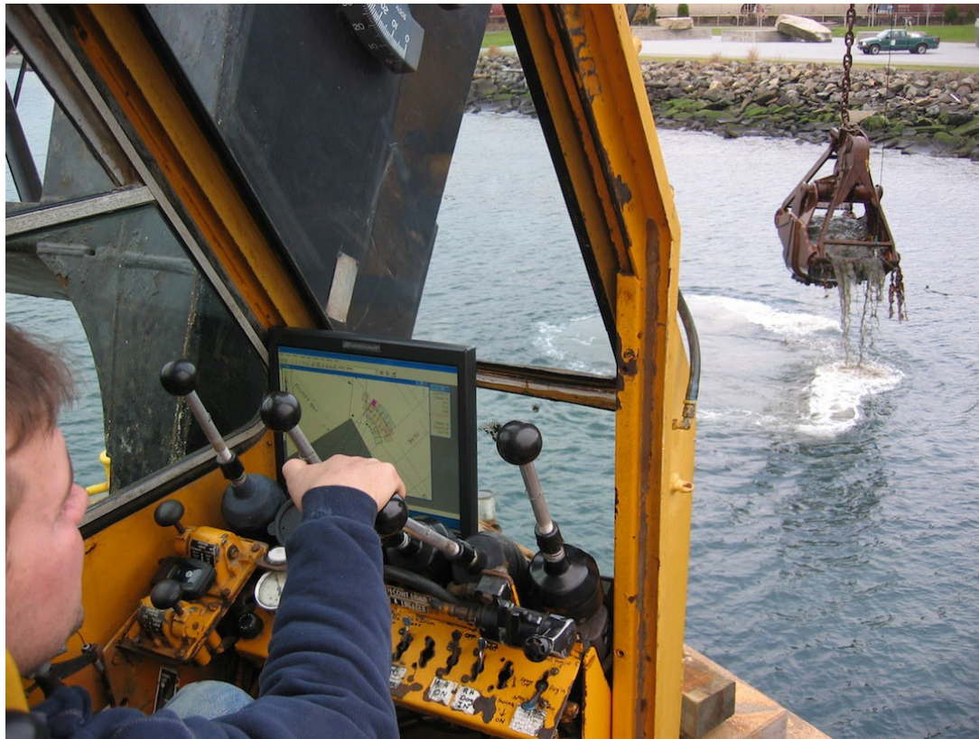
Open clamshell bucket example – debris in mud
