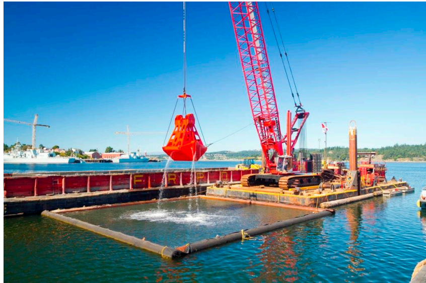
Derrick Barge with wireline bucket
